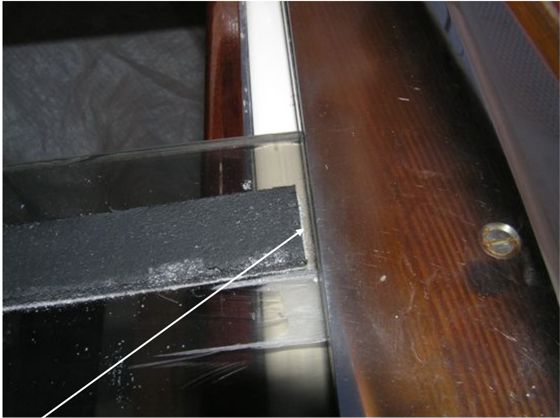
Gap at end of sealing strip
