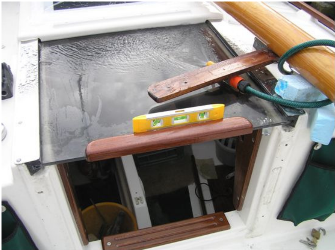
Testing to prove source of leaks
